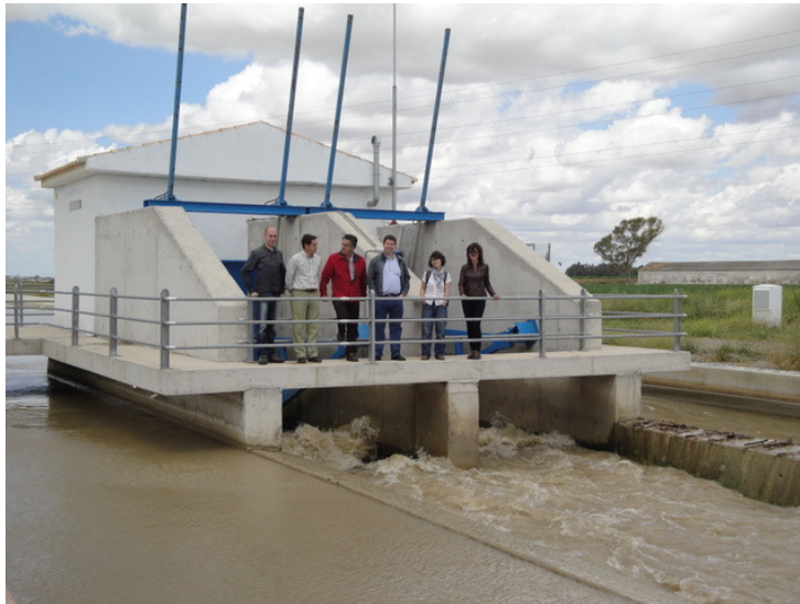
Figure 6. Two taintor gates with side weirs
