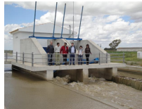
Two Taintor Gates with side weirs
